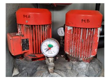
3~Mot 80A 7988891 N 022 /V 12 35772 357720 AF80/2C-11-ATB 400/230 \ YΔ 3,20/5,60 A 1,50 kW 2850 /min 50 Hz 0,85 CL F IP 55 EN 60034 K 160°C **B**2 CE Cent
